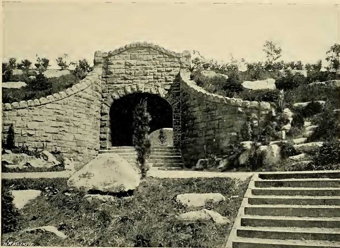
Tunnel under Main Road, Highland Park.
